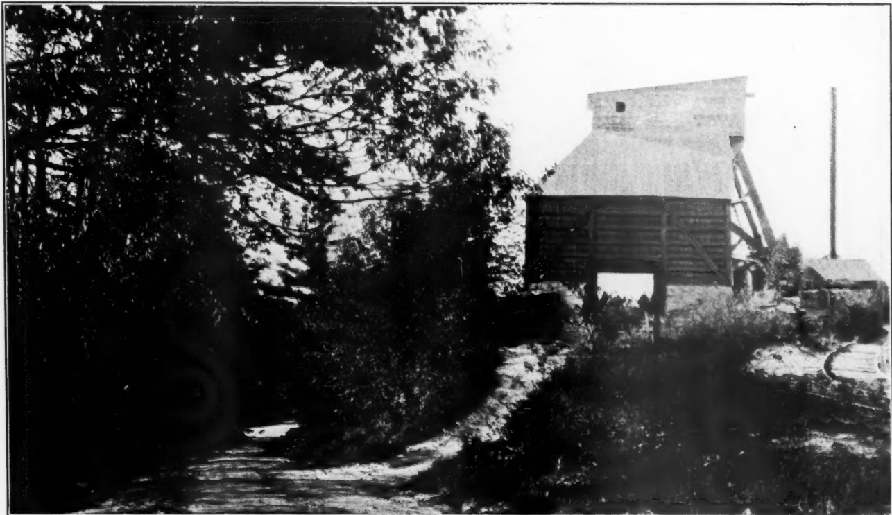
View of Crushing Plant, showing elevator and railroad sidings—one branch passing under the crushed stone storage bins and the other adjacent to the crusher.
